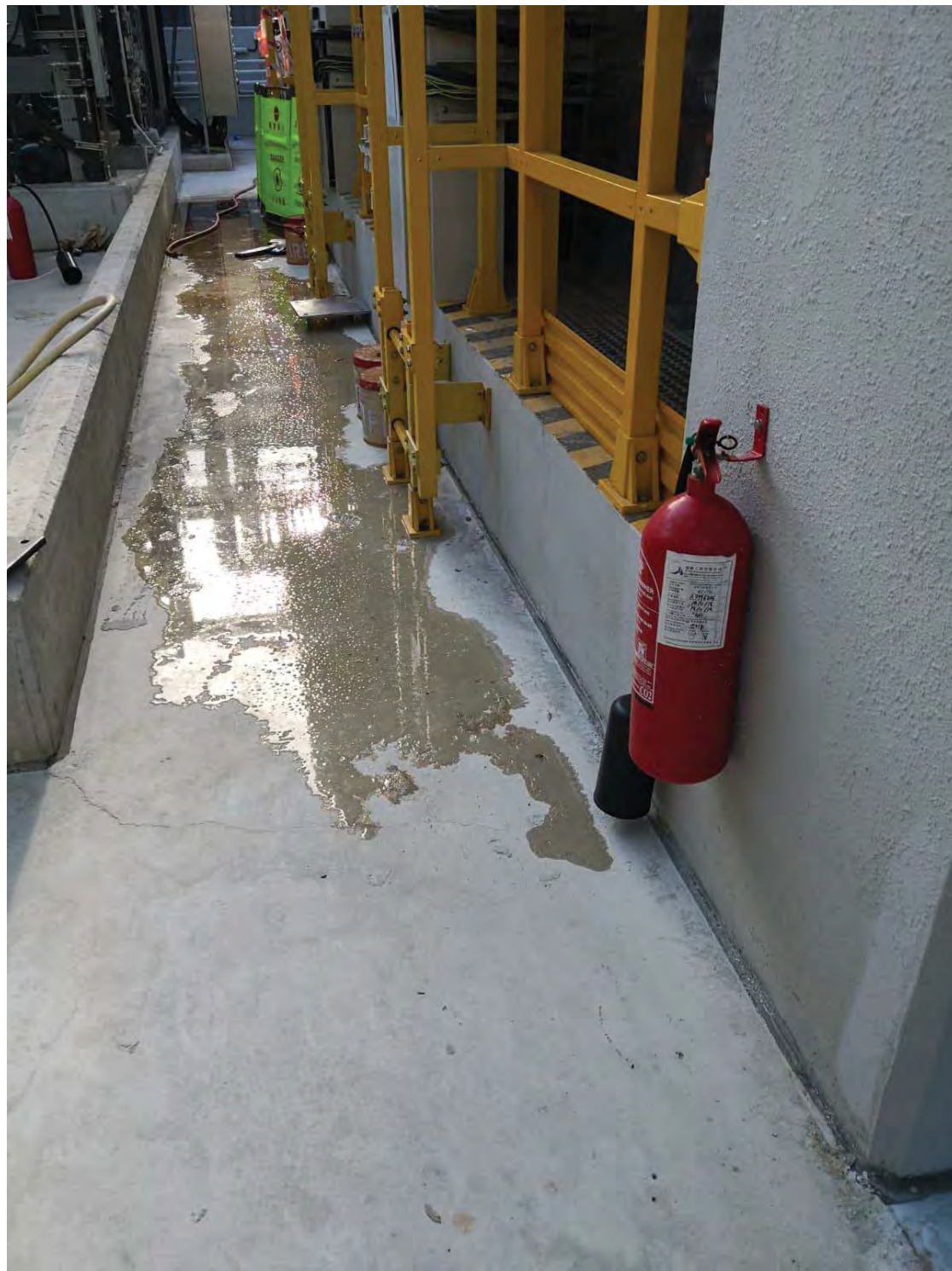
Chemical leakage observed on Building 1 roof.
